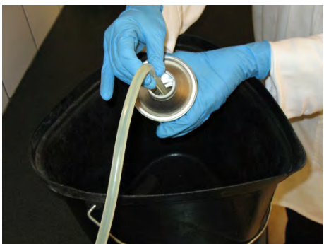
Connect the plastic or silicone tubing to the sampling valve. Make sure that the flange valve is closed. Open the transformer's valve. Operating the flange valve, rinse the flange and tube with at least 3 times its volume. Rinse the sampling tin by filling 1/3 with oil at least 3 times. Rinse the lid of the sampling tin
