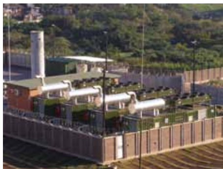
Durban solid waste landfill gas to electricity plant courtesy of Clarke Energy
